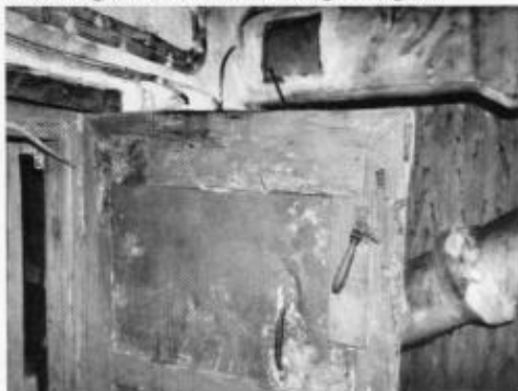
Heathfield Zero Station internal door showing closing handle and locking latch. A rubber gasket surround prevented generator fumes entering the main chamber. Air handling pipes can be seen in the background.
