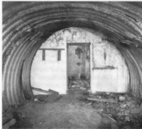
The main chamber of the Shipley Zero station looking towards the entrance shaft. This appeared to be in good condition when visited in 1997 but by March 1999 the chamber had collapsed. Photo Nick Catford
